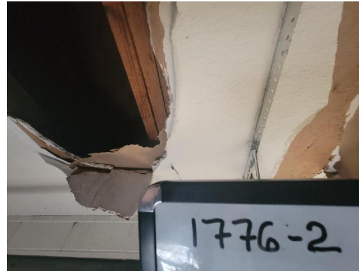
1776-2 Drywall/Joint Compound Typical Interior Walls/Ceilings
